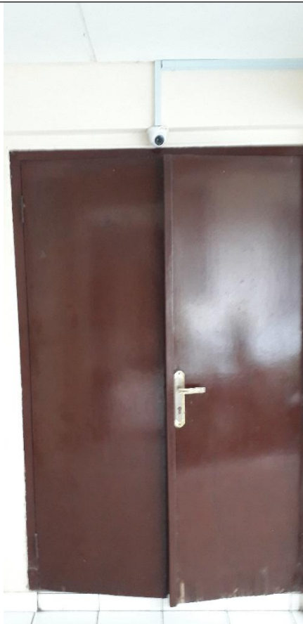
Cctv Area Lorong
